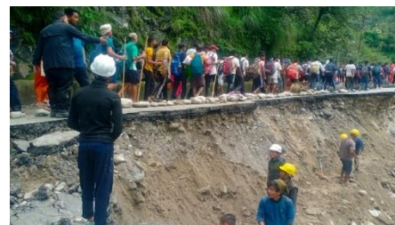
Pilgrims walk on the side of a washed-away trekking route to Kedarnath in Uttarakhand’s Rudraprayag district.
