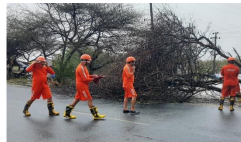
NDRF Team on road restoring work Source: Media
